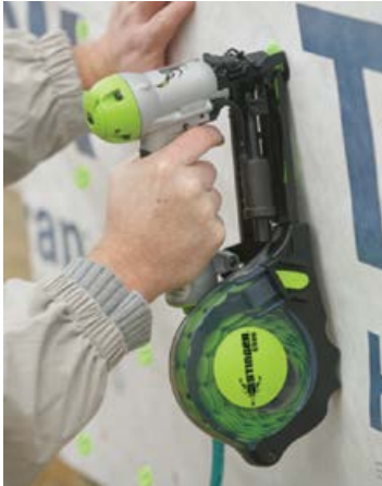
Pneumatic cap nailer that efficiently attaches building wraps to wood substrates.
