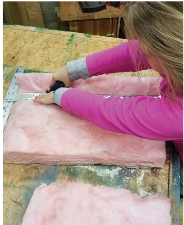
Cutting fiberglass insulation to fit between the wood and steel studs of the mini "hot box".
