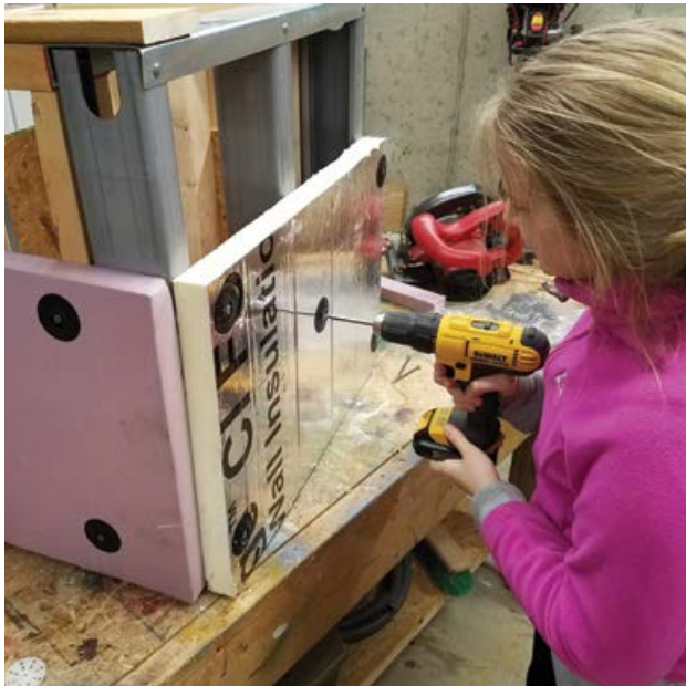
Attaching continuous insulation to wood and steel studs using thermally efficient Thermal-Grip washers and screws.
