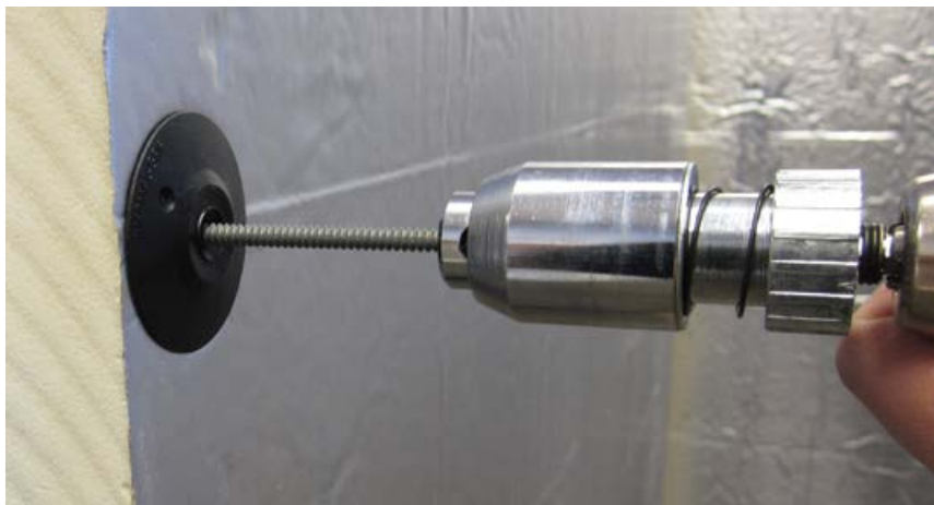
Chuck adaptors prevent screw wobble and overdrive of washers through rigid insulation.
